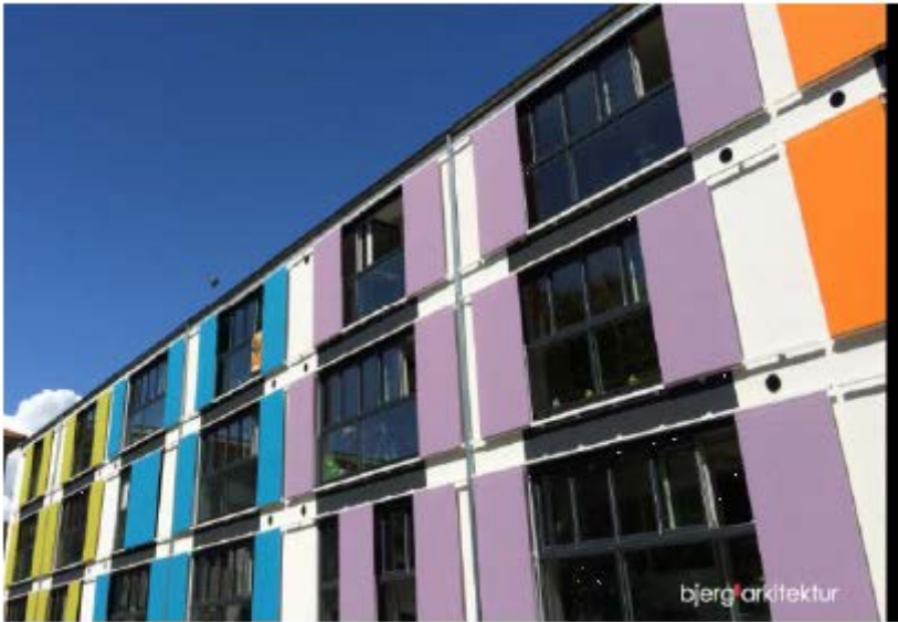
Apartment block after renovation
